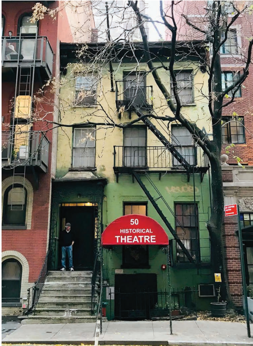
50 West 13 th Street, Greenwich Village. Photo: Village Preservation. The Jacob Day advertisement reproduced on the facing page is courtesy of Daytonian in Manhattan.
