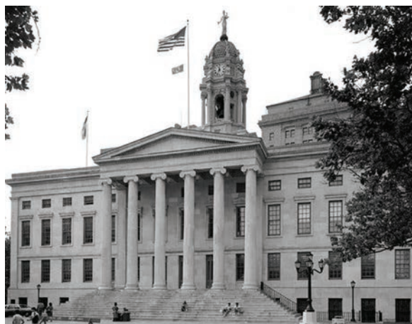
Borough Hall in Brooklyn in 1990. As the architect behind its restoration in the late 1980s, Mr. Conklin brought “intelligence and affection” to the project, the New York Times architecture critic Paul Goldberger wrote. Credit: Jack Manning/The New York Times.
