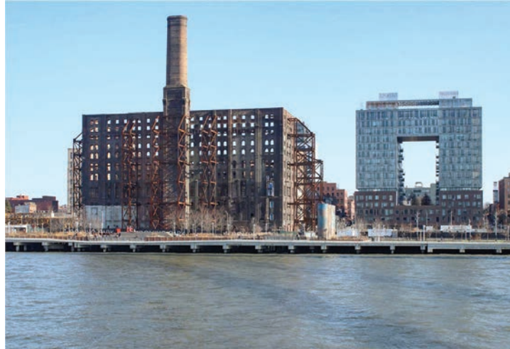
Under construction. Photo: Susan De Vries for Brownstoner.
