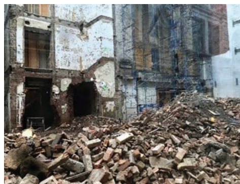
In 2021, reduced to a pile of rubble. Photo: Rick Stachura.
