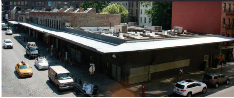
The former Gansevoort Market building in the Gansevoort Market Historic District. Photo: AM New York
