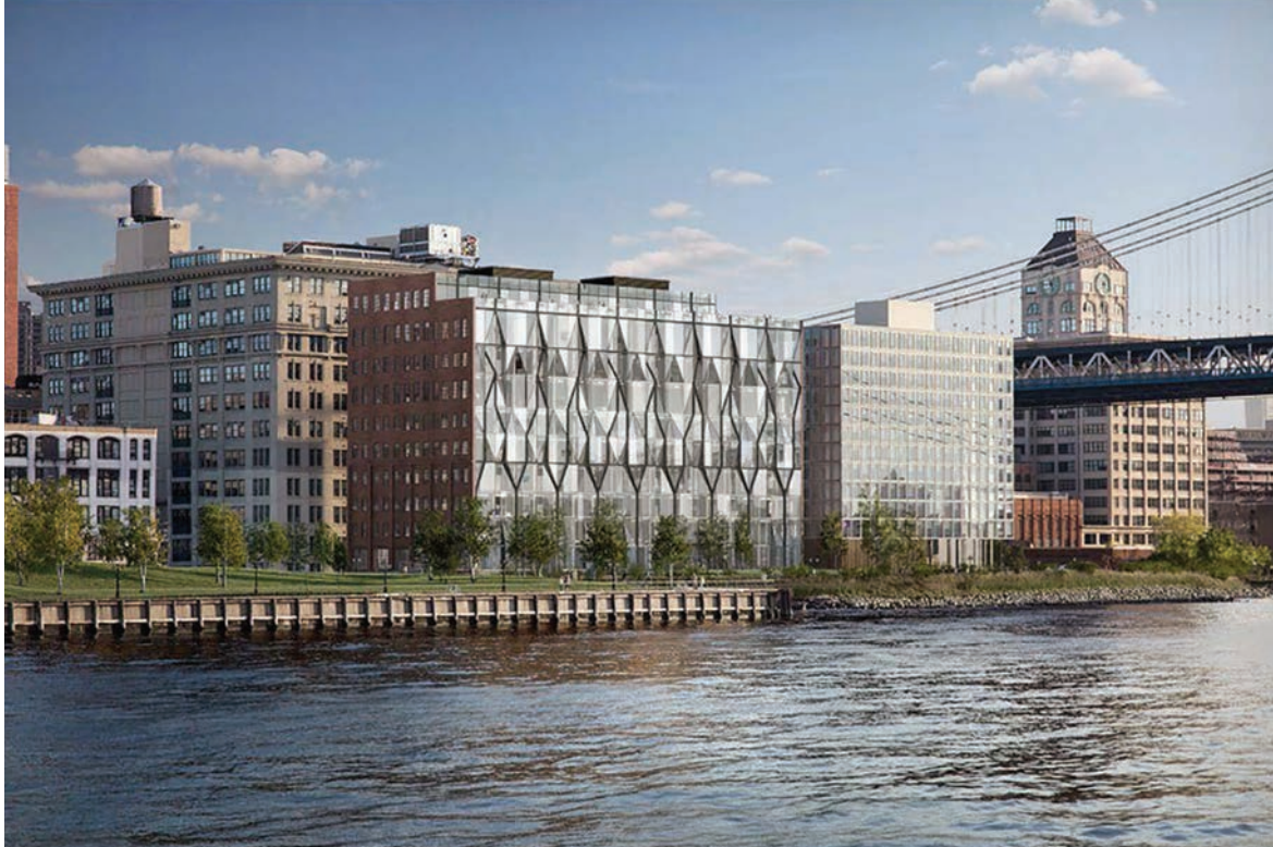
The river side of 10 Jay Street, said to recall crystals. of sugar. Image: ODA Architecture.
