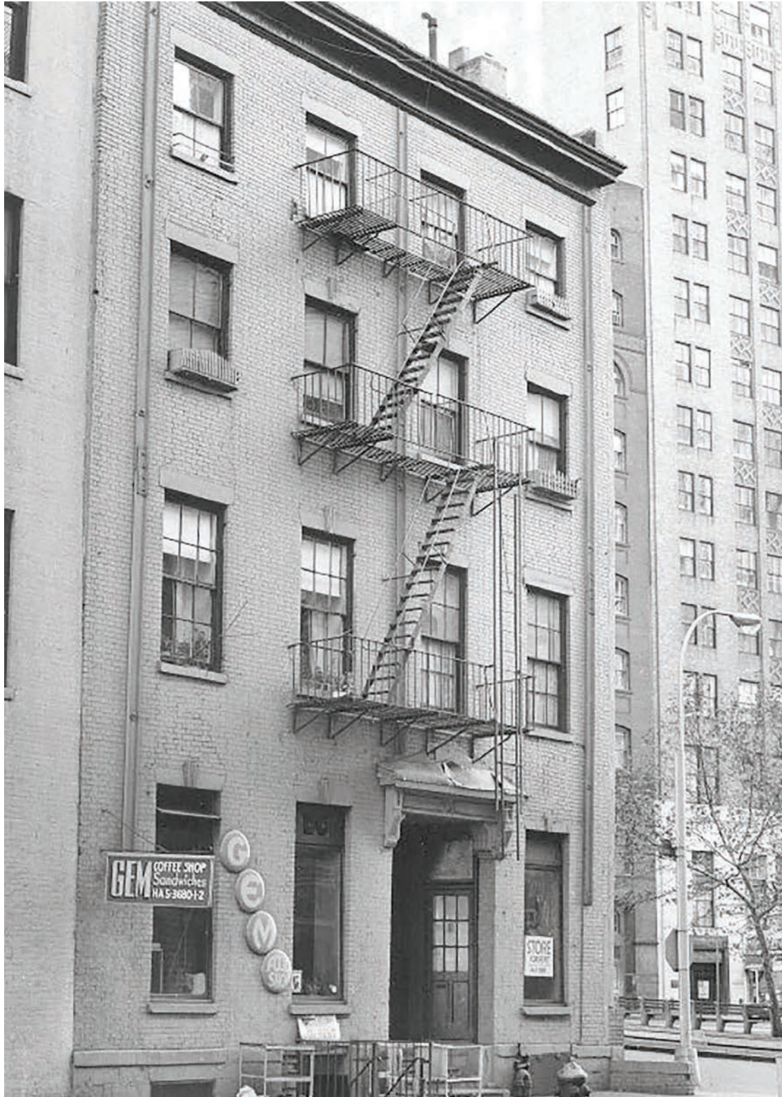
Before landmark designation, and thus before regulation provided by the de Blasio administration, the building at 67 Greenwich Street had survived for almost two centuries. It has now been radically rebuilt as part of a new development. Photo from Ephemeral New York.
