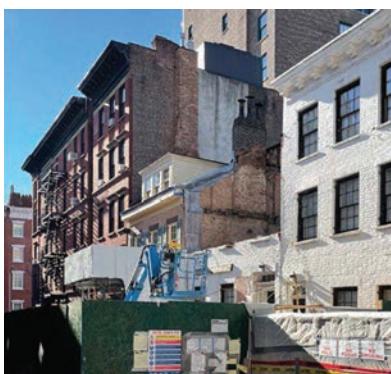
14 Gay Street demolition, ordered the Buildings Department. Photo: YIMBY.
