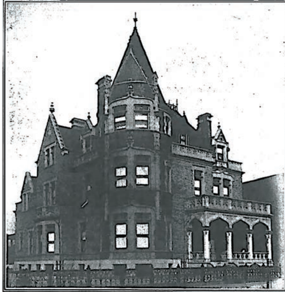
RESIDENCE OF MR. JACOB DANGLER, CORNER OF WILLOUGHBY AND NOSTRAND AVENUES. One of the most striking examples of the elaborately designed residences that are becoming an architectural feature of Brooklyn.
