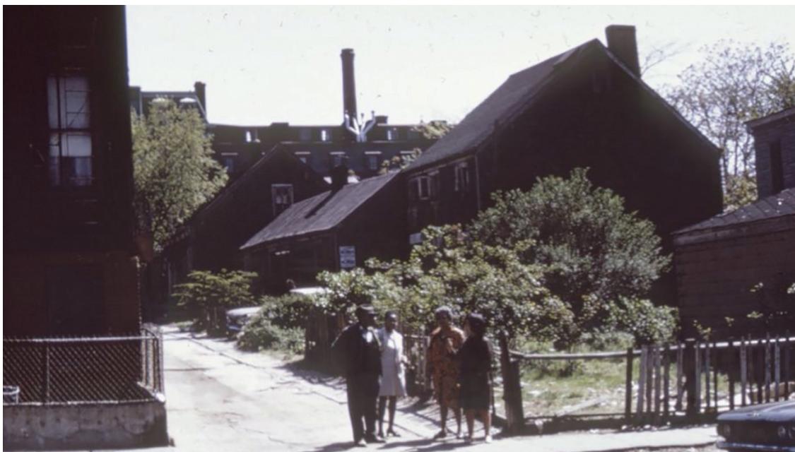
The Hunterfly Road Houses, 1706-1708 Bergen Street, before restoration. Photo: Landmarks Commission.
