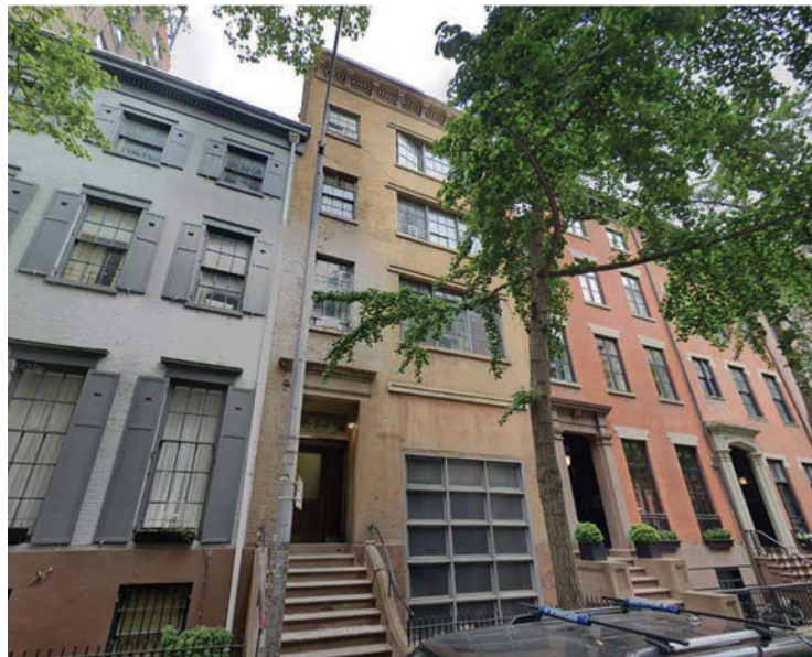
Before: two old rowhouses on East Tenth Street once converted into early 20th century artist's studios will now be one vast residence featuring a “great room.” Photo: Village Preservation.
