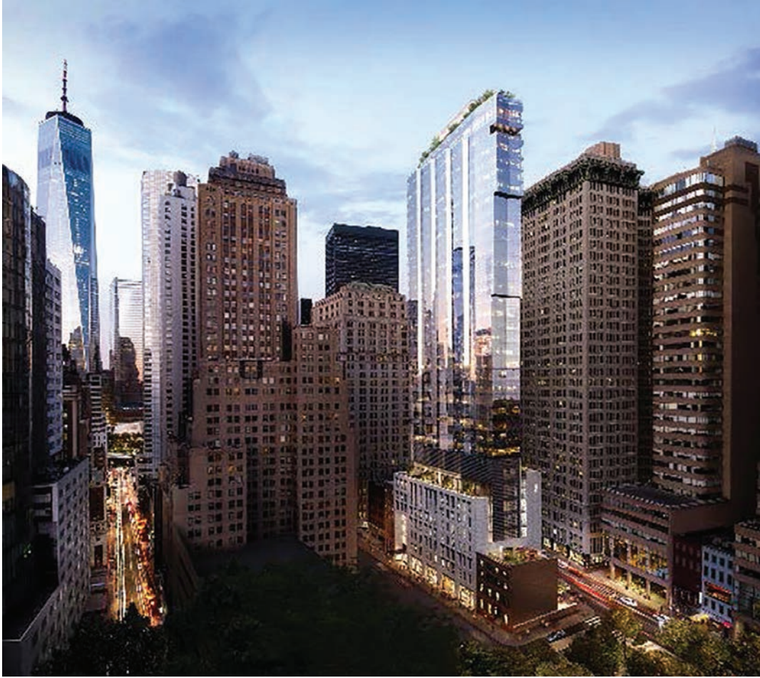
The new building at 77 Greenwich Street, known as The Jolie, shown attached to the roofless remains of the individual landmark, the former 67 Greenwich Street, dating from 1810. Rendering: Landmarks Preservation Commission.
