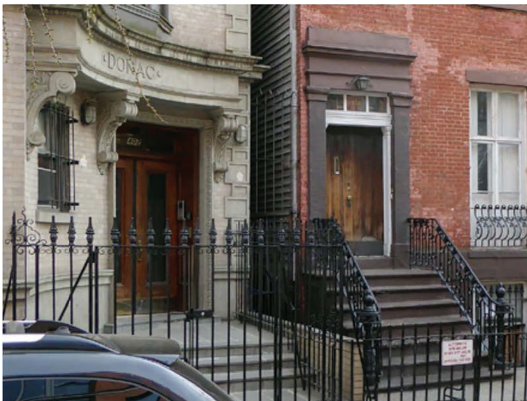
The oldest house in Chelsea, dating from 1830, 404 West 20th Street is endangered by administrative actions of the LPC under Chair Srinivasan. An approval was issued allowing the demolition of the side and rear walls, the roof and the interior for an enlargement, preserving nothing but a fraction of the street façade. The house is now for sale. Photo of the original structure showing the original horsewalk at left: David Holowka, Architakes.
