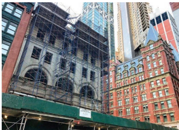
Photos below: Demolition. Courtesy of Rick Stachura, notesonnewyork.net.
