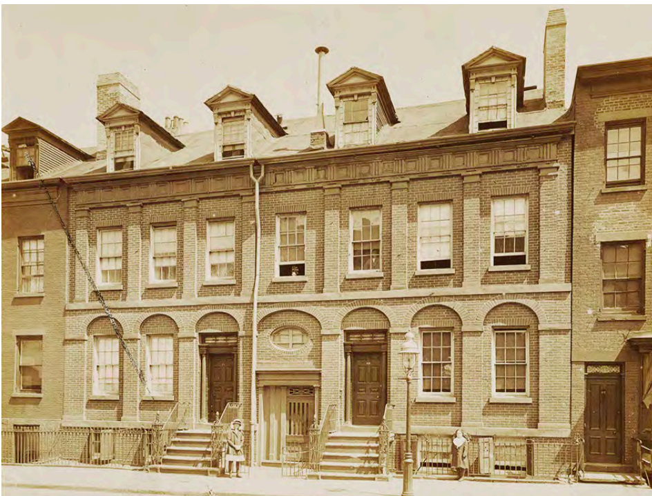
69 & 71 Charlton Street, between Varick & Hudson Streets, 1913; Courtesy of the Public Design Commission
