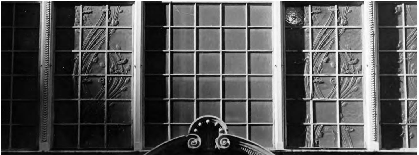
René Lalique windows on the third floor of the Coty Building, c. 1984; Courtesy of the Anthony C. Wood Archives
